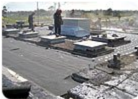
Workers carefully flash the antenna bases.
